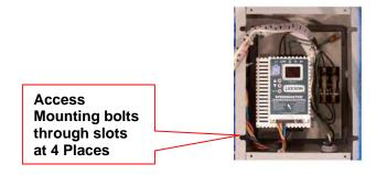
**15.** Attach the conduit elbow to the bottom of box by removing the nut, slipping the fitting through and then installing and tightening the nut.
